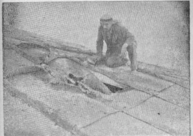
Bomb Damage in 1948
